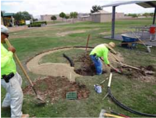
Adding the Base Material
