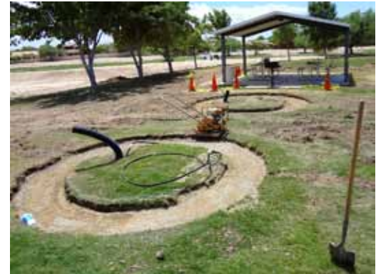
Compacting the Base Material
